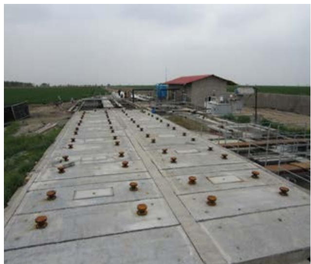
Image No. 30: Anaerobic basins at Salehi and Saffari (Chaltasian) dairy farm.
