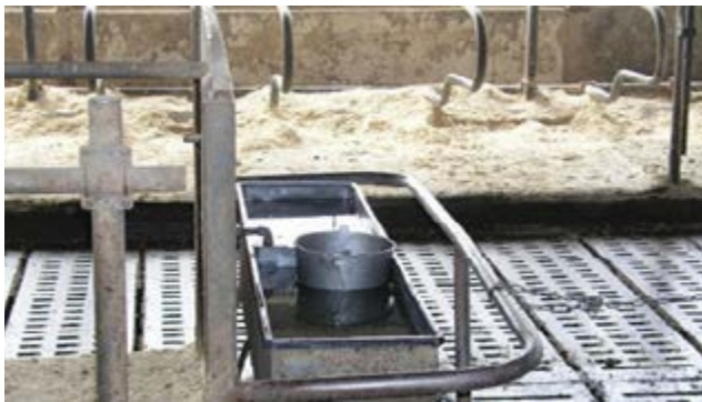
Image No. 3: Grooved concrete flooring
