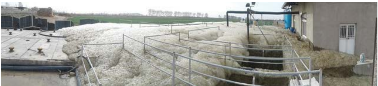
Image No. 34: Production of foam by bacteria in biological treatment plants.
