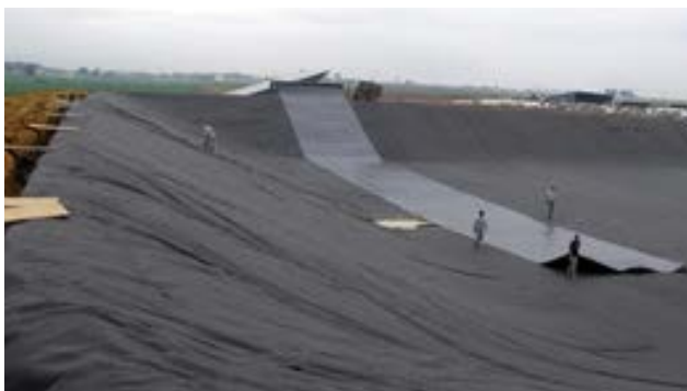
Image No. 28: Stages of constructing liquid manure storage facilities.
