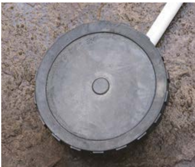
Image No. 33: The blower and diffuser samples used in Salehi and Saffari (Chaltasian) dairy farm.
